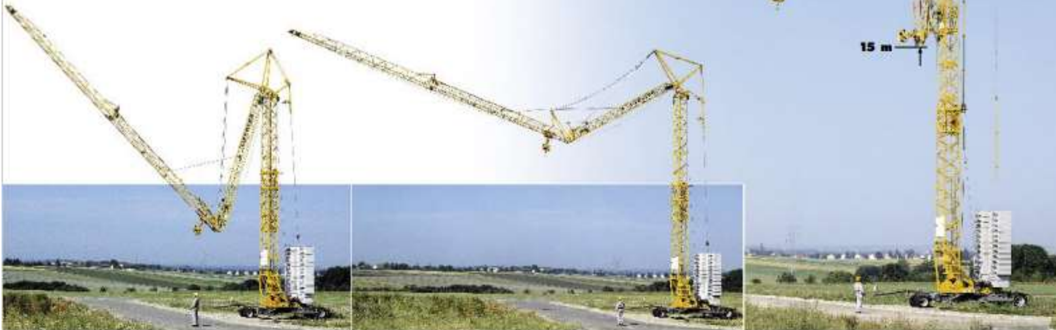
Aerial jib mounting without tower sections.
